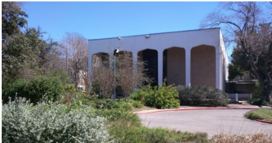
Congregation Beth Israel • Travis County Boilers • Chillers • Window Film • BAS Controls Assessment: $450,000 • Annual Savings: $40,000
